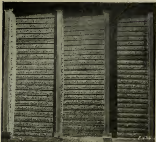
"SELF-SENTERING" REINFORCEMENT IN THE STAIRCASE AT DRURY LANE THEATRE (see p. 353).
